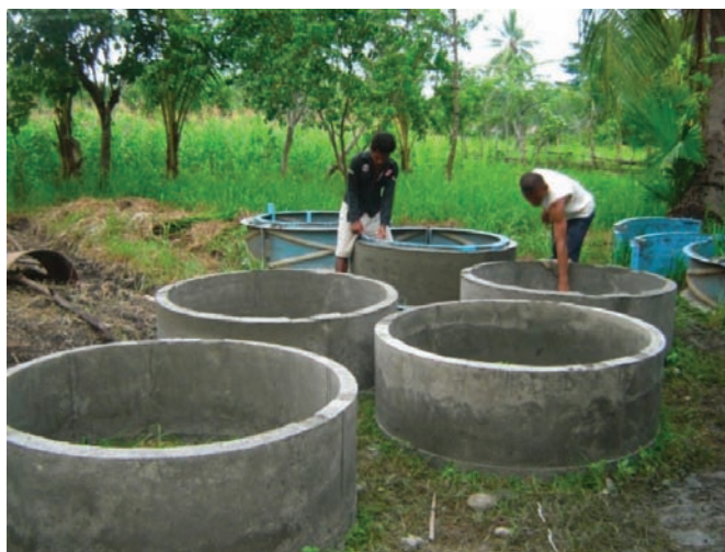
Photo 2: Preparation of concrete rings for construction of wells
