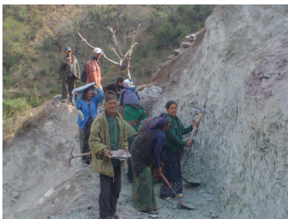
Photo 4: A worker group widens a track using simple tools
