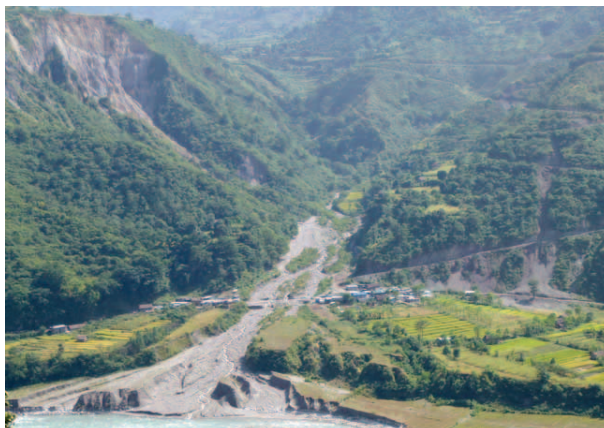
Photo 2: Settlement encroachment along roads in hazard-prone areas should be prevented
