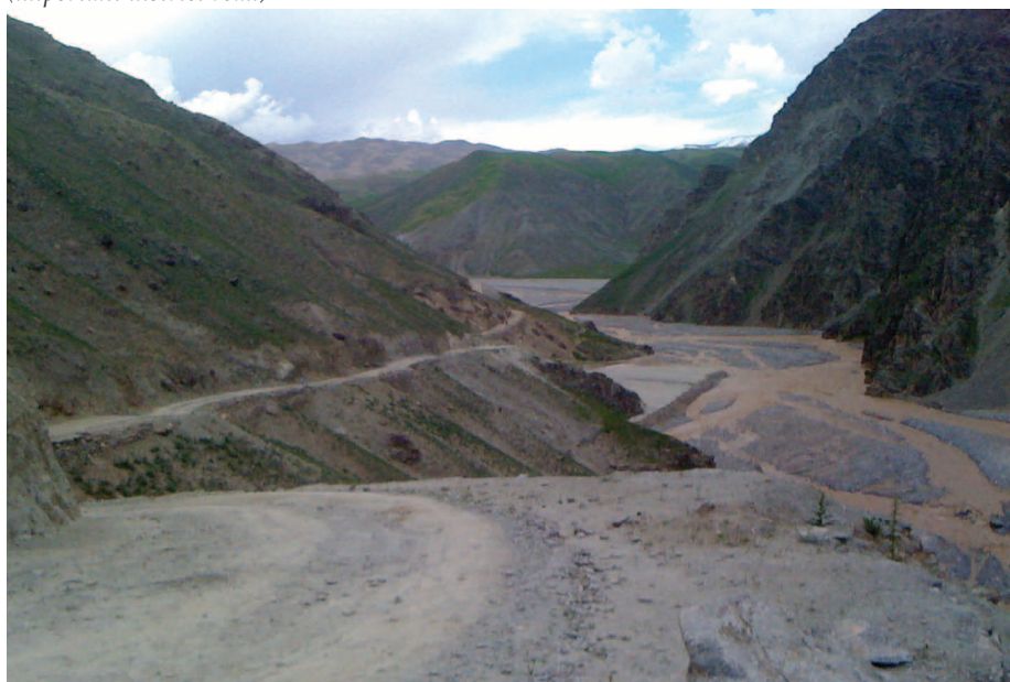
Photograph 1: Example of labour intensive backbone project (important district road)
